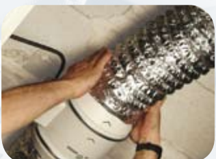
Connect the ducts
