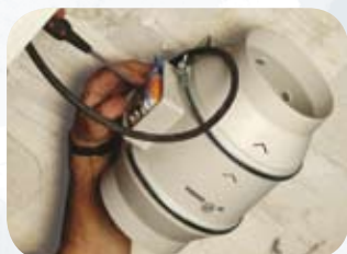
Carry out the wiring connections
